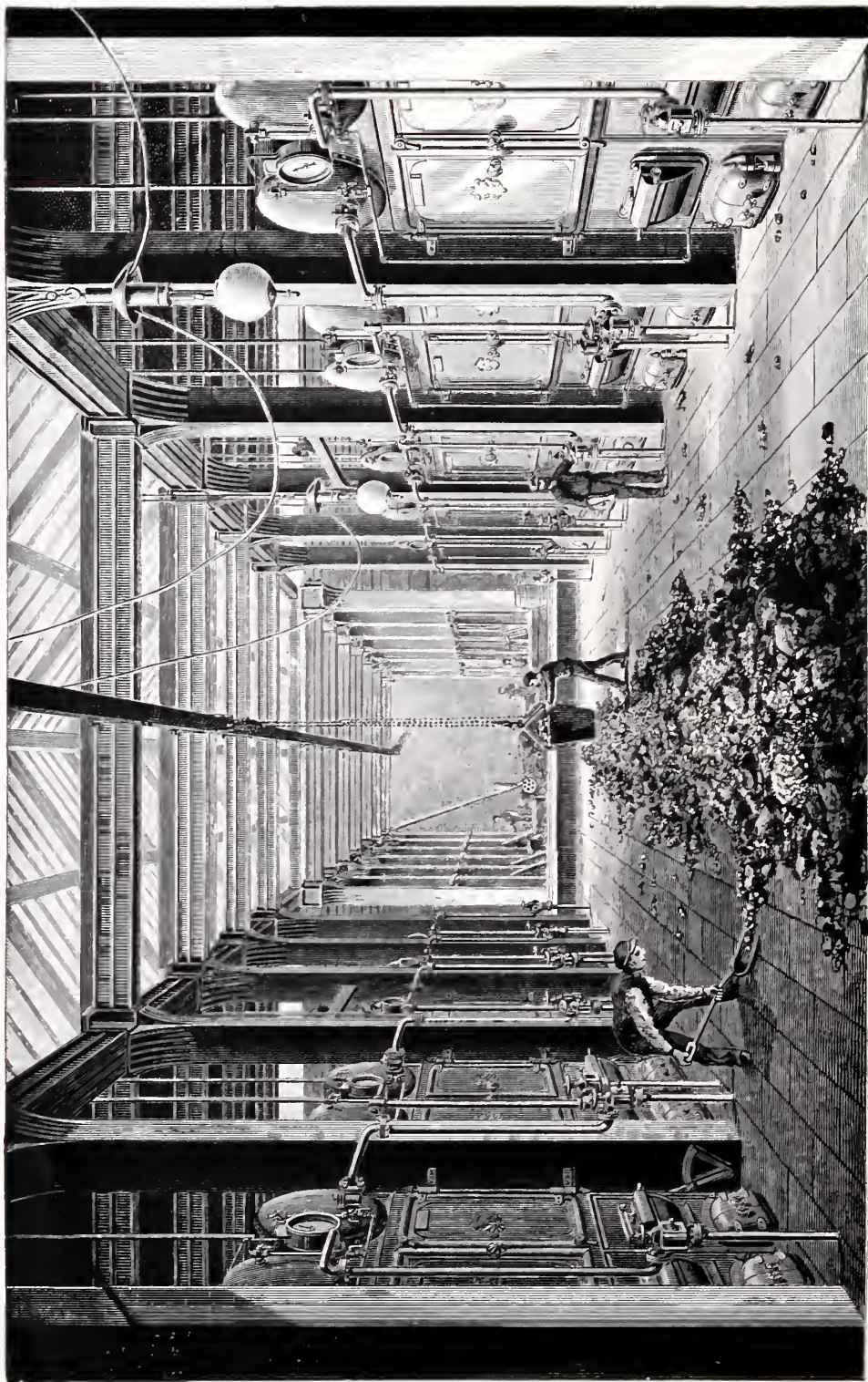
Babcock & Wilcox Boilers at Deptford Station of the London Electric Supply Corporation, Limited; 25 Boilers, 12,000 indicated H. P., with Compound Engines. Erected 1888-9. To have 120,000 H. P. when completed.
